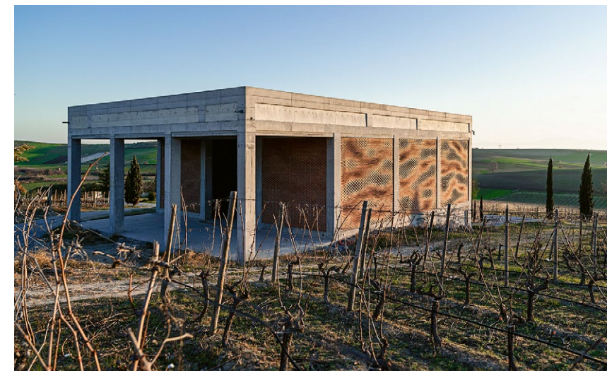
A wine cellar at the foot of Mount Olympus: the technology creates visual effects in the brickwork.
